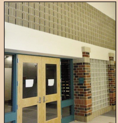
Onekama Elementary School Location: Onekama, MI CMU Producer: Michigan Certified Concrete
